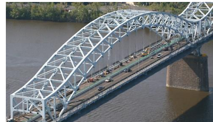
Figure 1: Aerial photo of a single Arrigoni Arch
